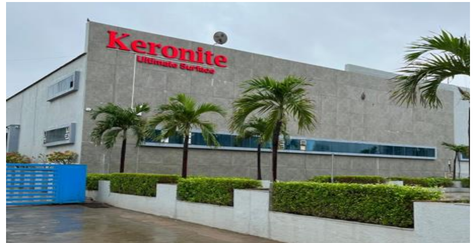
Keronite Tiles. Gujarat
