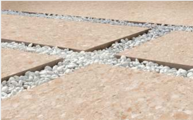
Laying on Gravel
