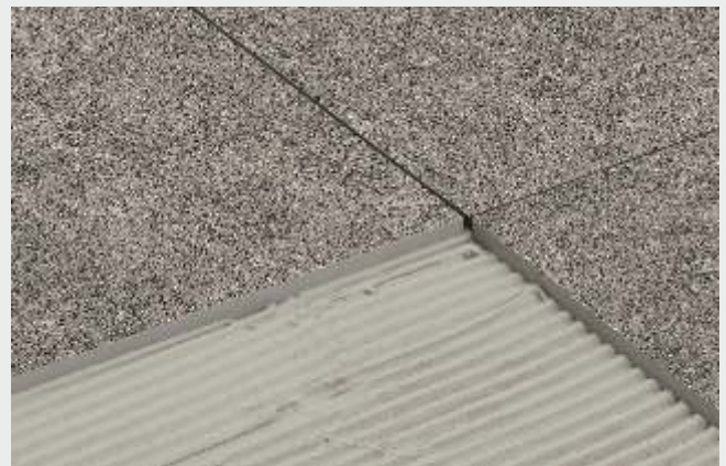
Laying with Adhesive
